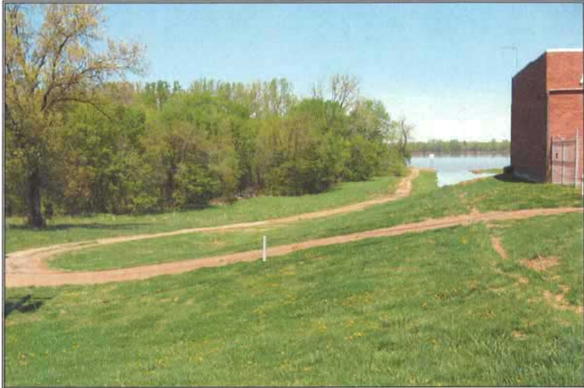
Photograph 1: Facing north along the proposed new access road, from the southeast property corner on the floodwall. A total of 0.17 acre of wooded habitat will be cleared to the left of the existing path along the very edge of the existing tree line. Paducah Riverfront Boat Launch. April 2, 2007.
