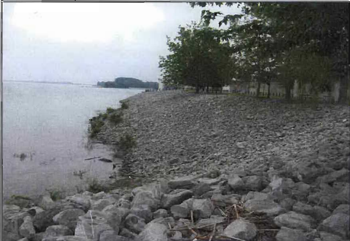
Photograph 3: Facing upstream in the area of the proposed Schultz Park expansion. The existing Schultz Park is located above the riprap bank to the right. Paducah Riverfront Development Phase 1 / Transient Dock. May 14, 2008.
